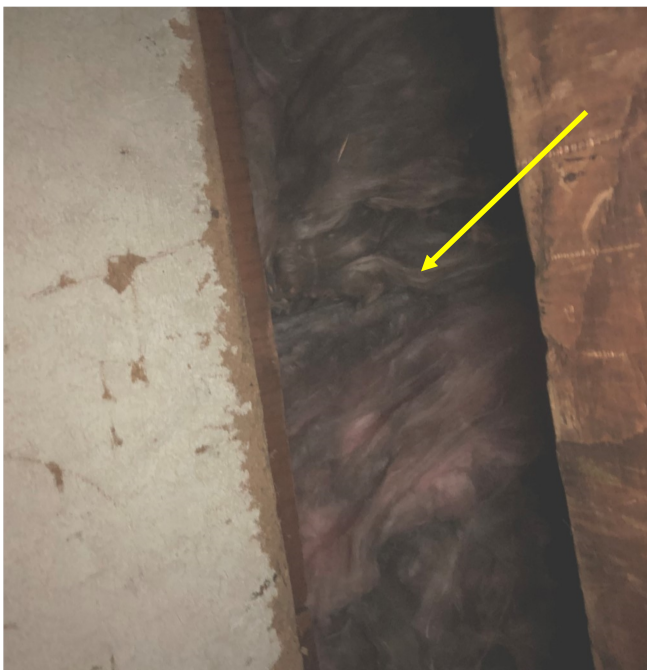
Dark areas indicate thermal bypasses to the outside.
